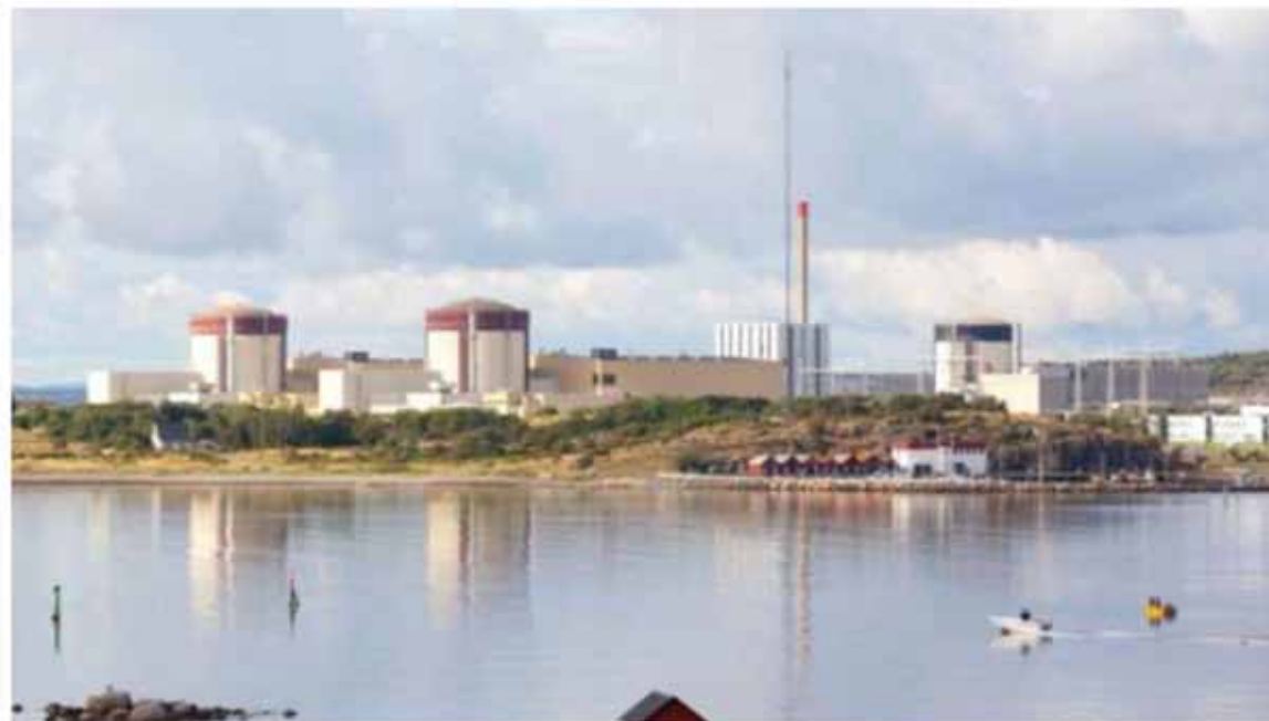
The four-unit Ringhals plant (Image: Vattenfall)
